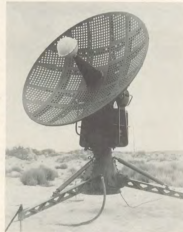
Weather Radar Antenna
